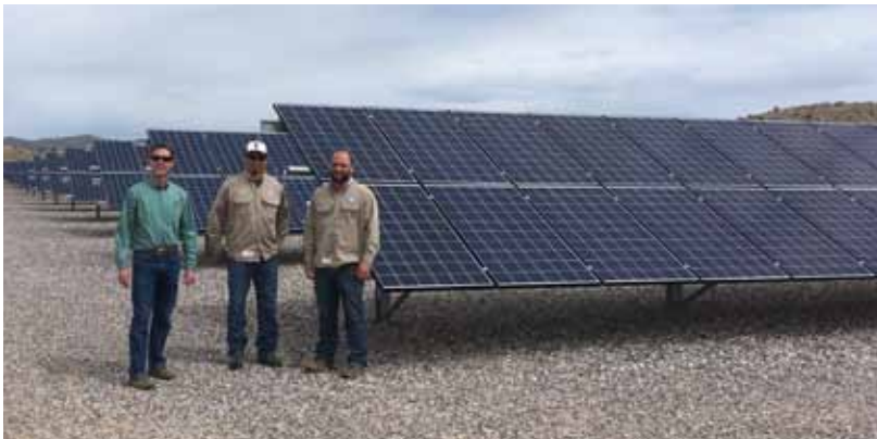
Photo (Left): In 2018, the Governor's Office of Energy staff inspected previously completed projects, including the Lincoln County Power District's community solar project seen here. (source: GOE)
