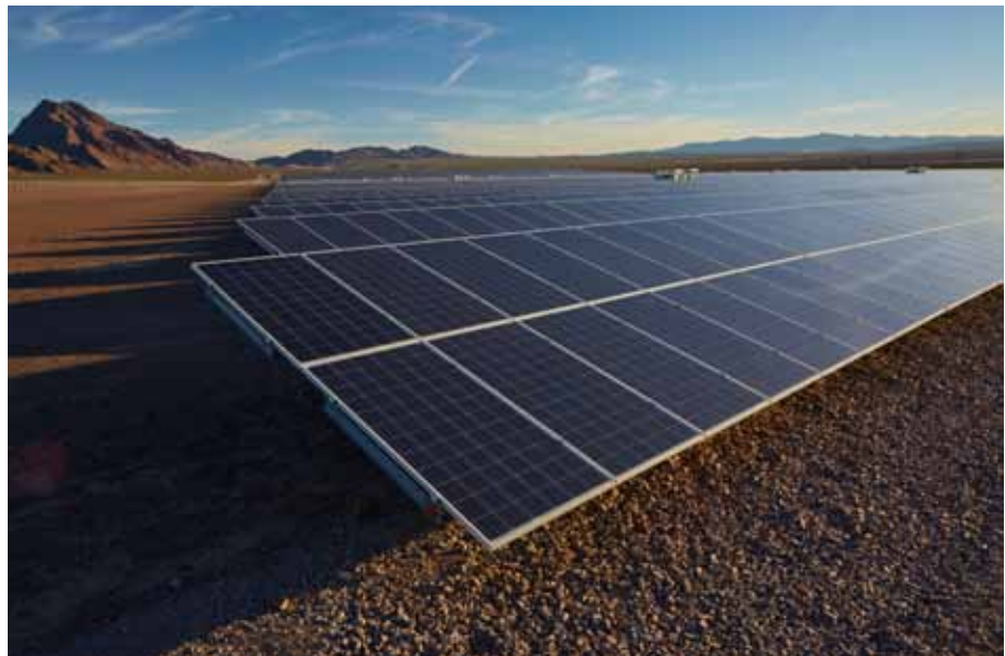
Photo: Sempra's Copper Mountain Solar Project (Source: Sempra).
