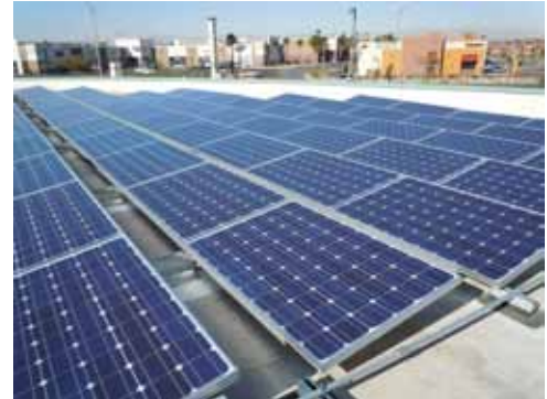
Photo (Above): Solar installation on the Henderson DMV building (source: GOE).
