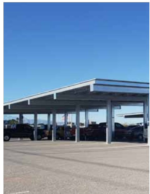
Photo (Right): Solar install over parking structure for the City of Las Vegas - West Yard (Source: City of Las Vegas).
