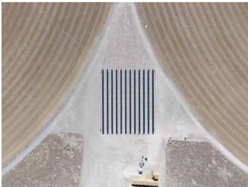
Photo (Left): Aerial view of PV installation at Railroad Valley Farms (Source: Railroad Valley Farms).
