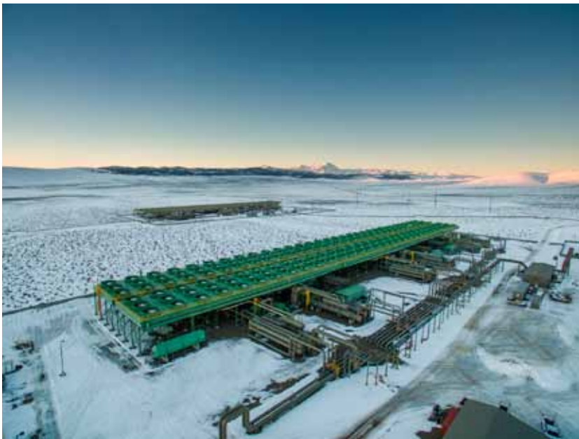
Photo: Ormat's McGinness Hills geothermal power plant (Source: Ormat).
